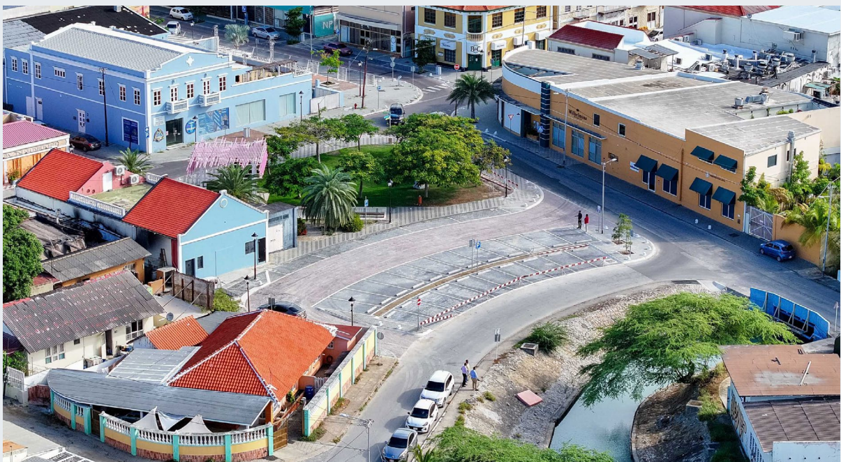
Revitalization of Lagoon parking lot area. Credit: Aruba Department of Nature & Environment.
